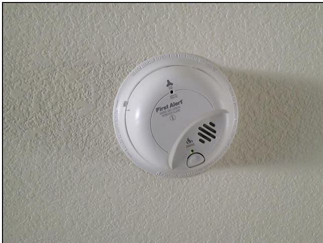
7.7 Item 1(Picture) Combination CO and Smoke detector
