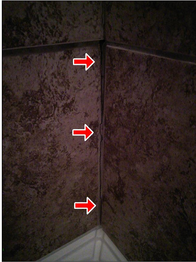
6.1 Item 1(Picture) Basement Shower Crack
