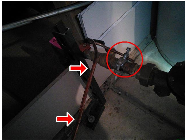
7.1 Item 4(Picture) Water System Grounding
