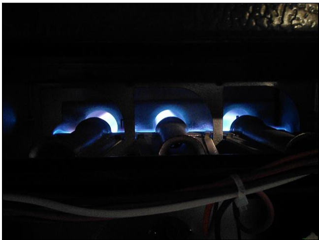
8.0 Item 2(Picture) Goodman Furnace Ribbon Burners in Operation
