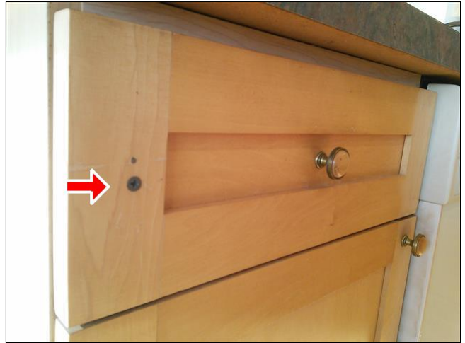
4.4 Item 7(Picture) Non standard drawer repair
