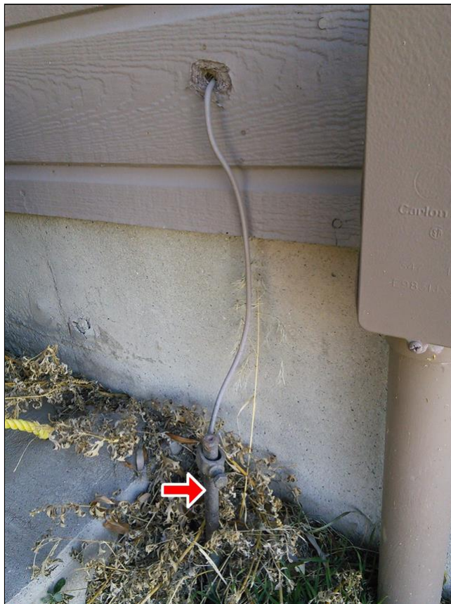
7.1 Item 4(Picture) Driven rod grounding system.
