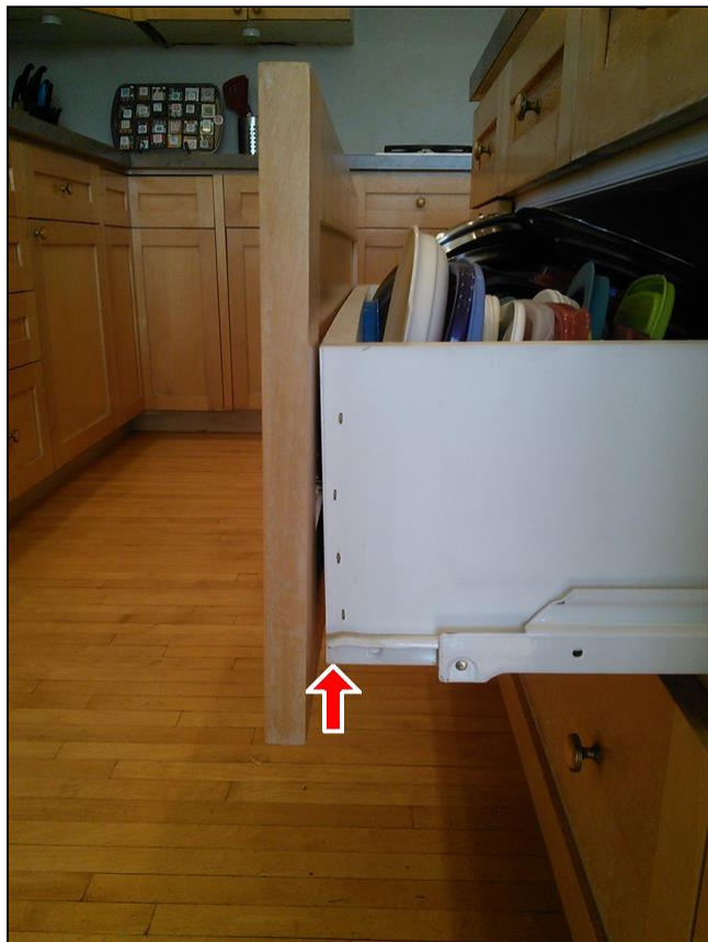
4.4 Item 8(Picture) Warped and loose drawer front
