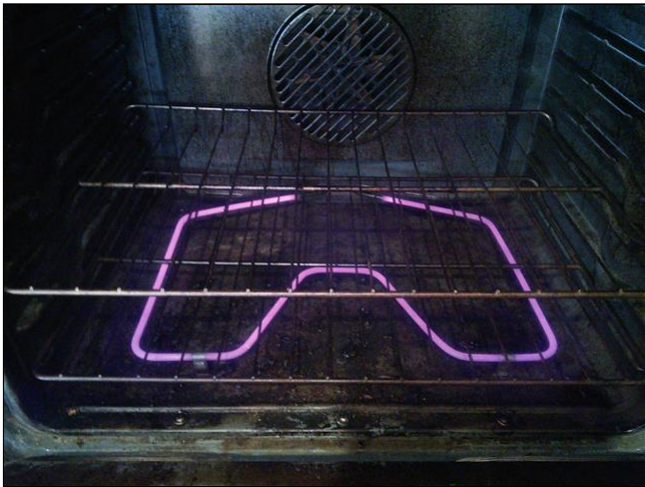
10.1 Item 8(Picture) Lower oven bake element
