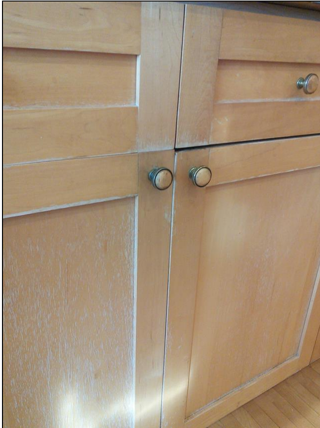
4.4 Item 6(Picture) Damaged finish
